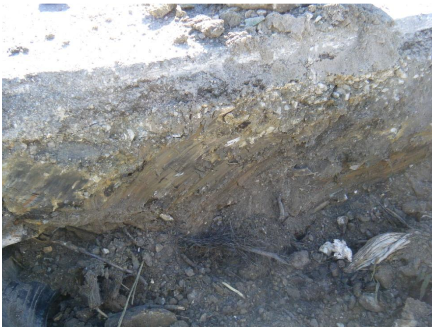
Photo 2 : Side of Pit Wall
