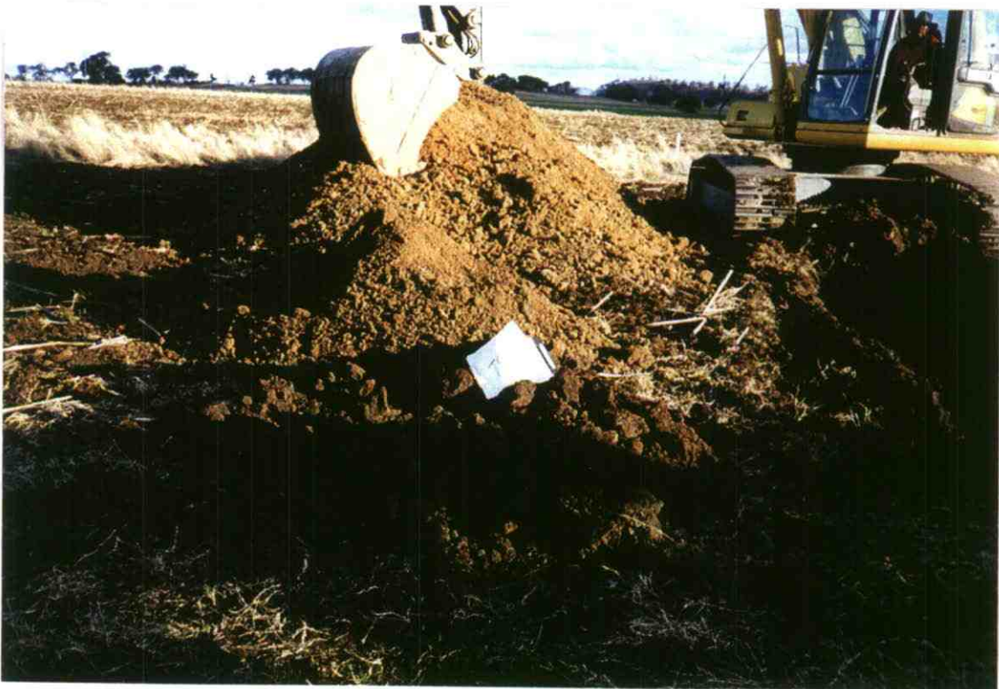
Plate 8: Excavated material from TP3
