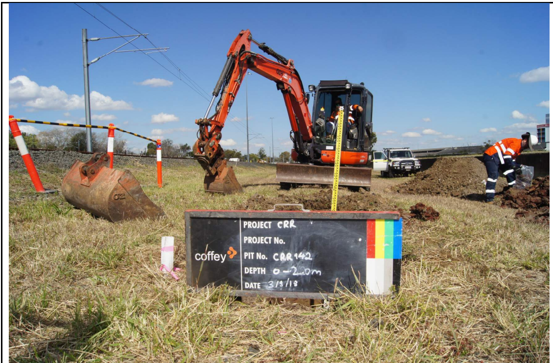
Photograph 2: Test pit site.
