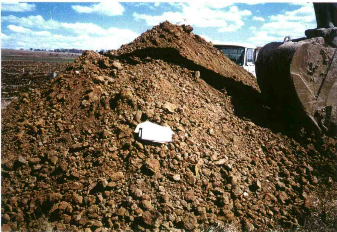
Plate 14: Excavated material from TP5
