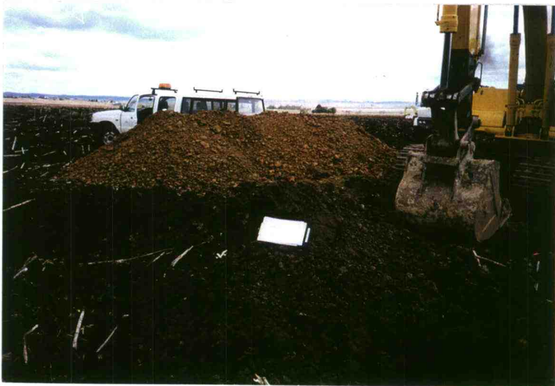
Plate 2: Excavated material from TP1
