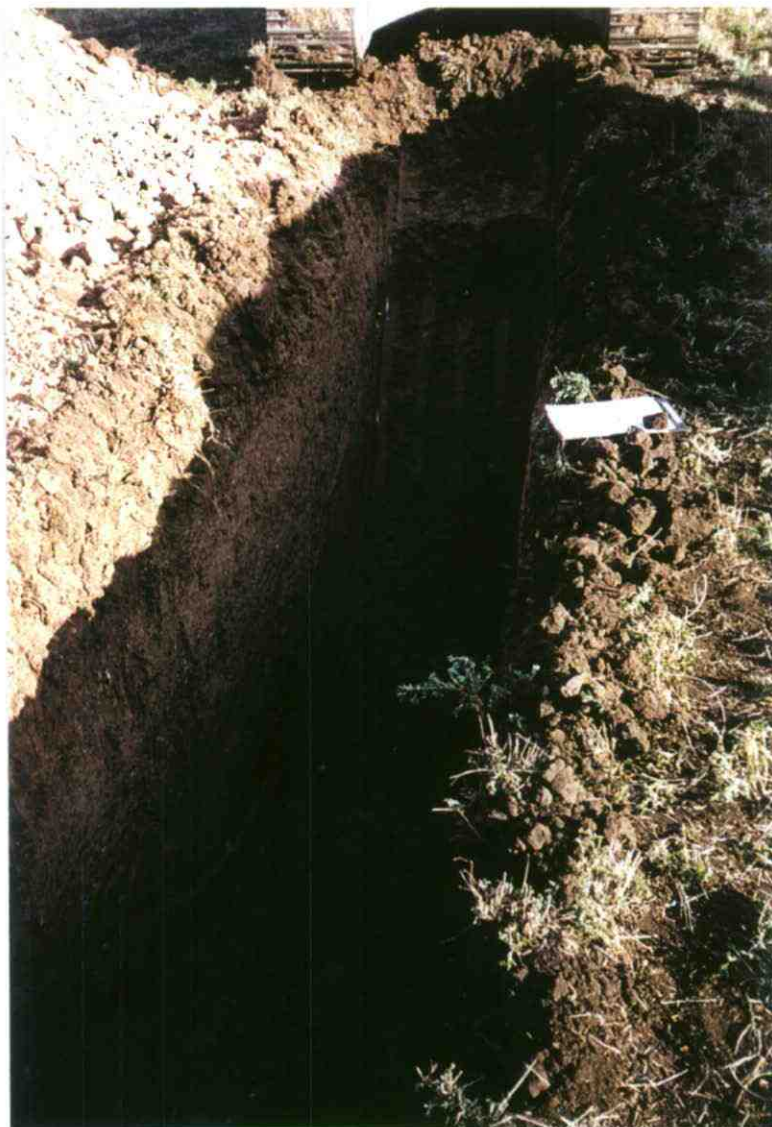
Plate 32: View inside TP18
