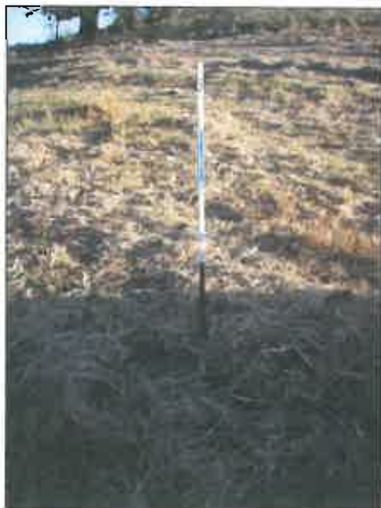
Site before excavation
