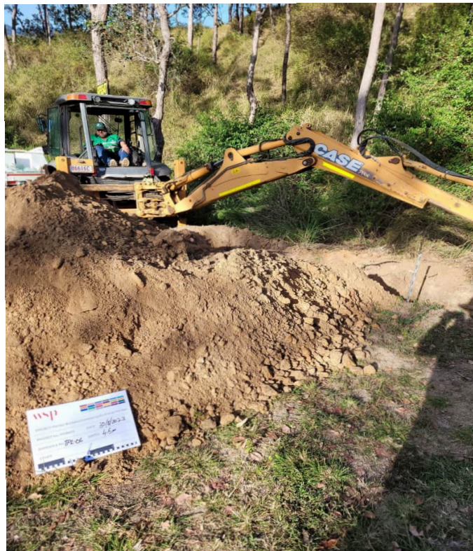
TPL-06 - 2 Depth Range: 0.00 m - Test pit excavated spoil
