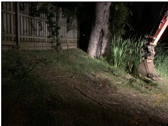
Testpit length and depth retracted due to telstra cable
