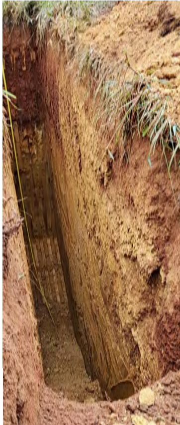
TPUA-06 - 1: Test pit excavation
