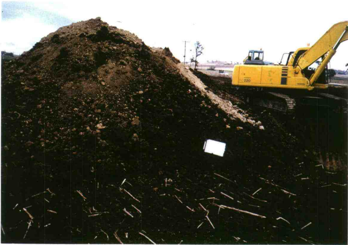
Plate 37: Excavated material from TP20
