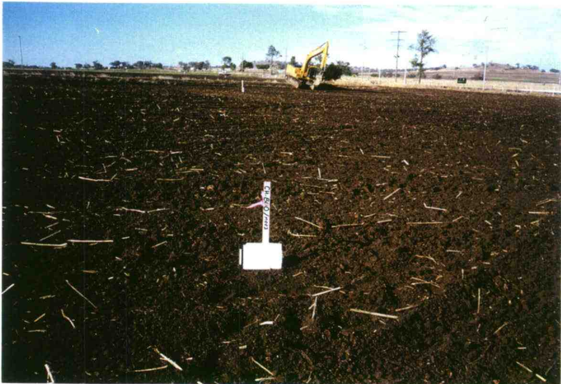
Plate 36: Site view of TP20
