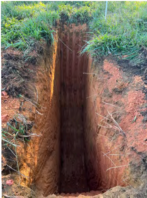
TPUA-04 - 1: Test pit excavation
