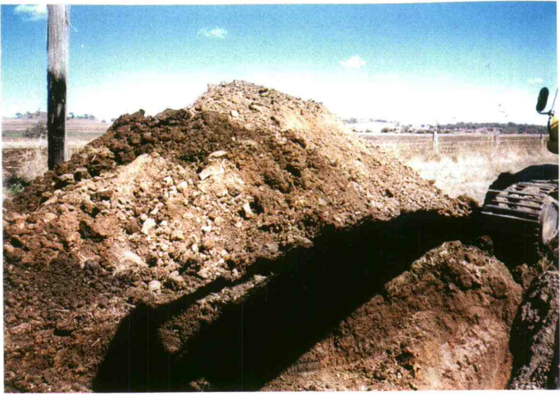
Plate 11: Excavated materials from TP4
