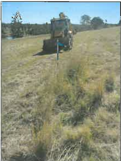
Excavation terminated at 4m Site before excavation
