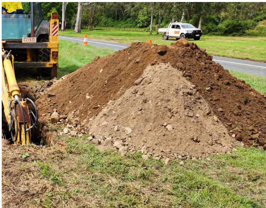
TPL-09 - 2: Test pit excavated spoil
