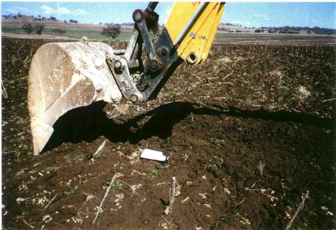
Plate 4: Site view of TP2
