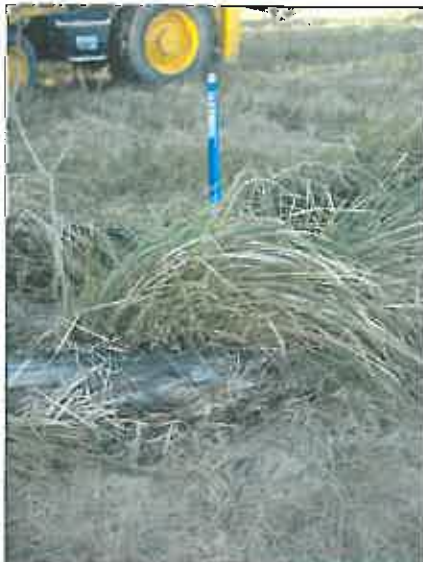
Site before excavation
