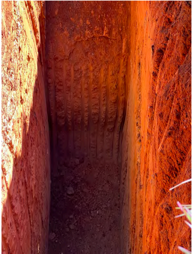
TPUA-21 - 1: Test pit excavation
